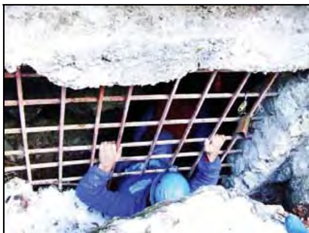
Figure 7. Upstream entry. Figura 7. Intrarea amonte.
